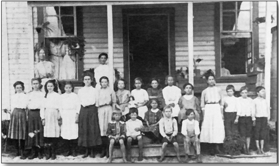
The Alva Consolidated School (c. 1900), located along the Caloosahatchee River.
