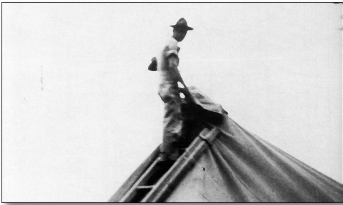
Soldier wiring a tent with electricity.
